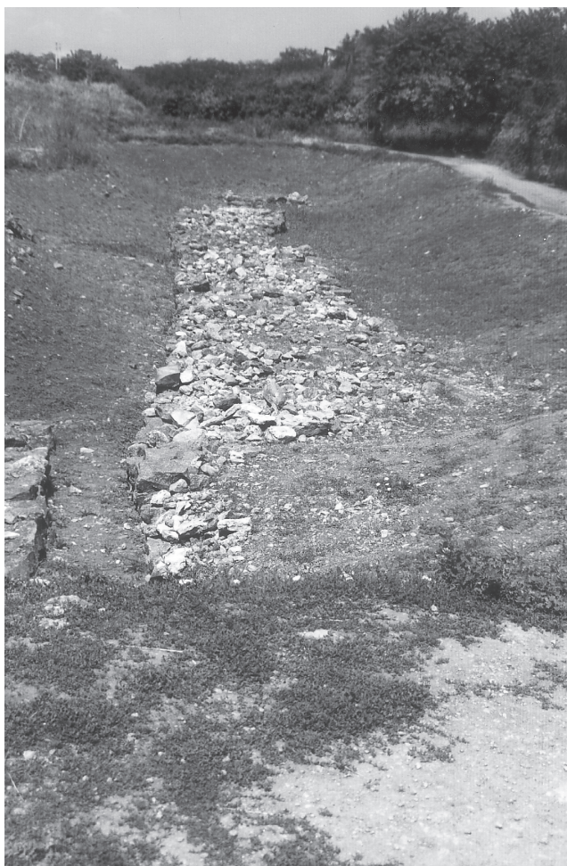
4. Defensive wall in the trench IX
