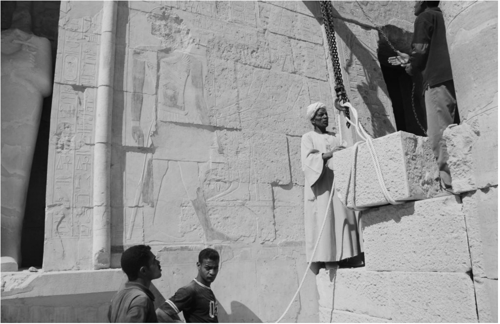
2. Dismantling the blocks of the Ptolemaic Portico wall covering the southern (left) scene placed close to the Granite Portal leading to the Main Sanctuary of Amun-Re. (Phot. M. Jawornicki).
