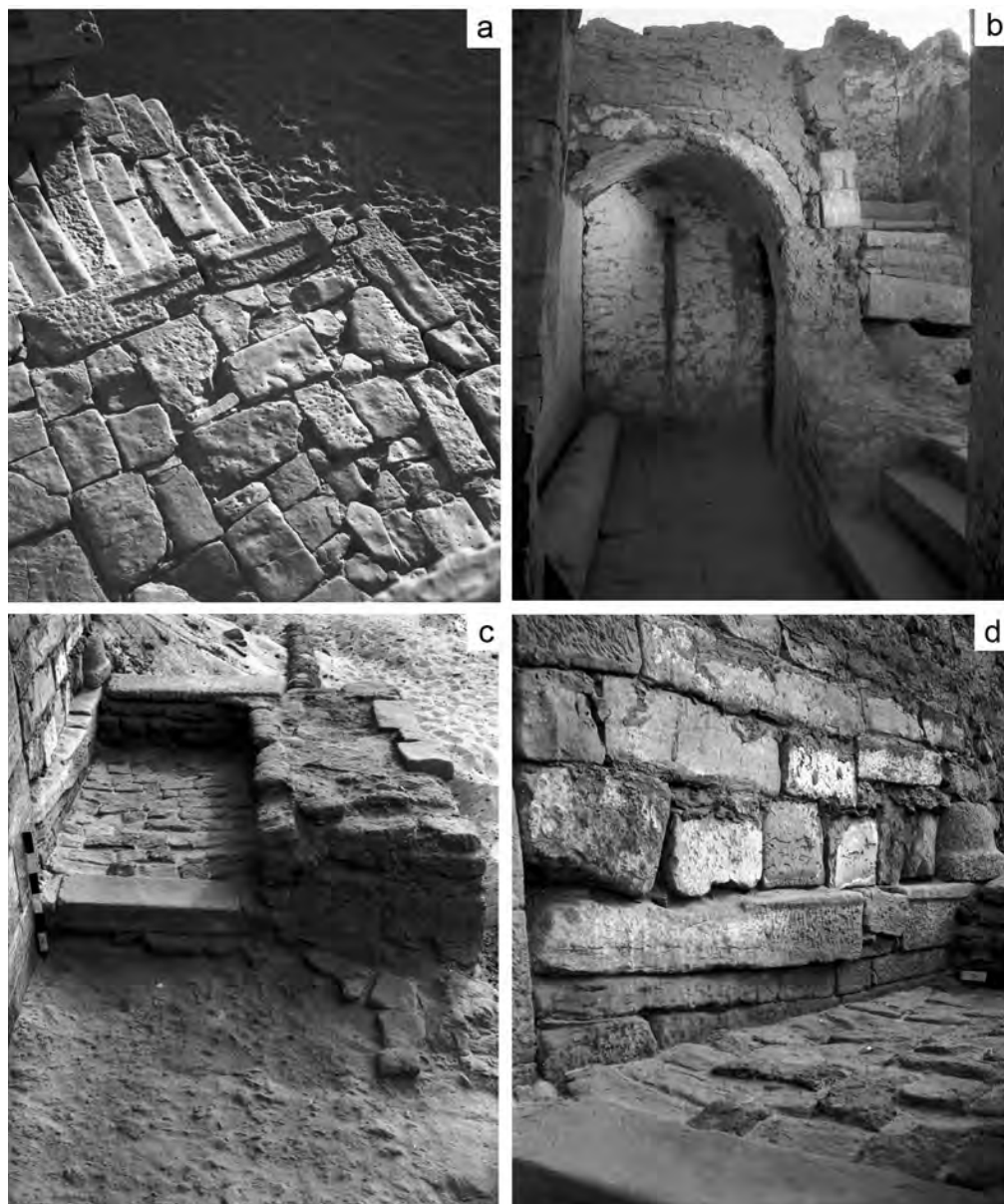
11. Area of the porch, architectural details: a. paving of the entrance platform; b. interior of the late twelfth-century staircase built on the porch seen from the north; in its construction a base and a granite block with carved channels on sides are visible; c. paved rectangular structure adjoined to the entrance platform from the western side, seen from the north; d. the entrance platform edge and the paving of the rectangular structure, seen from the north-west; note the wear and tear step on the edge and a capital embedded in the staircase wall (a-b. Phot. M. Niepokólczycki; c-d. Phot. T. Biniewski © IKŚiO PAN).
